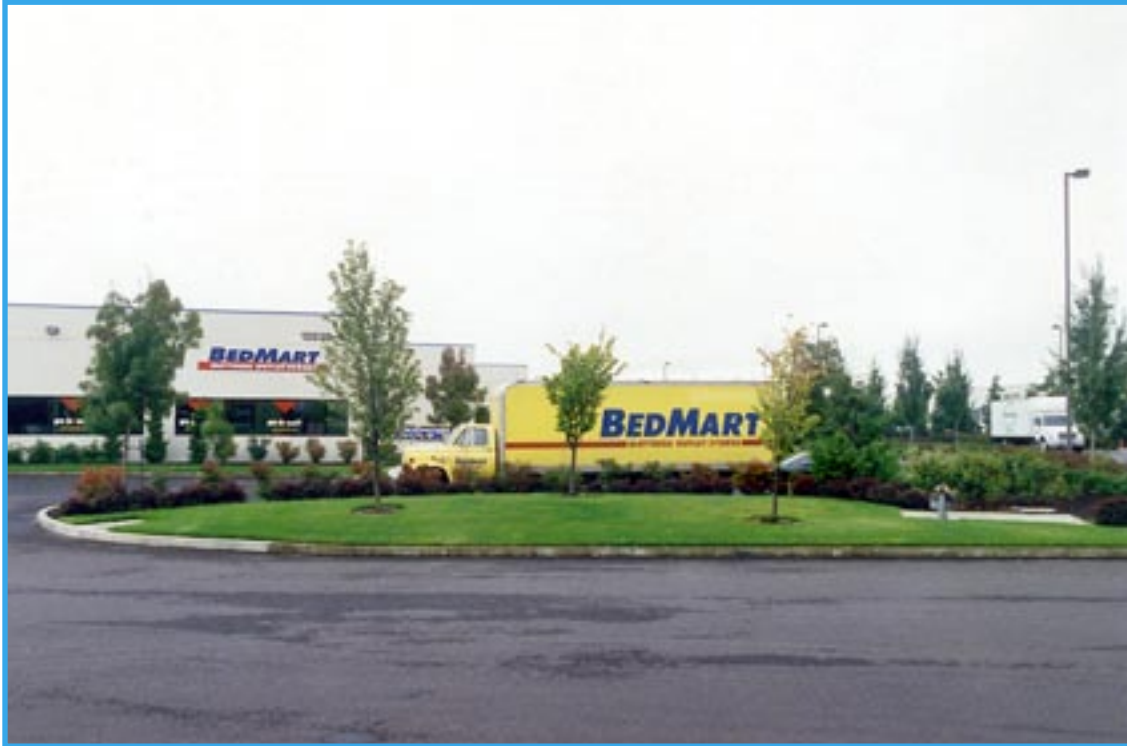
Looking East at Competition Space and Signage
